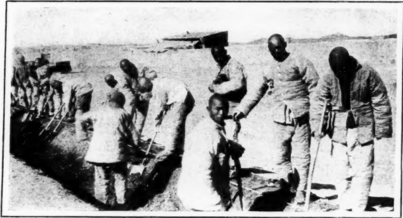
Feng's soldiers digging irrigation ditches
